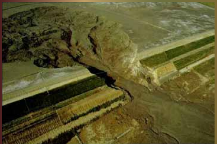
Aznalcóllar, Spain tailings dam rupture, April 25, 1998
