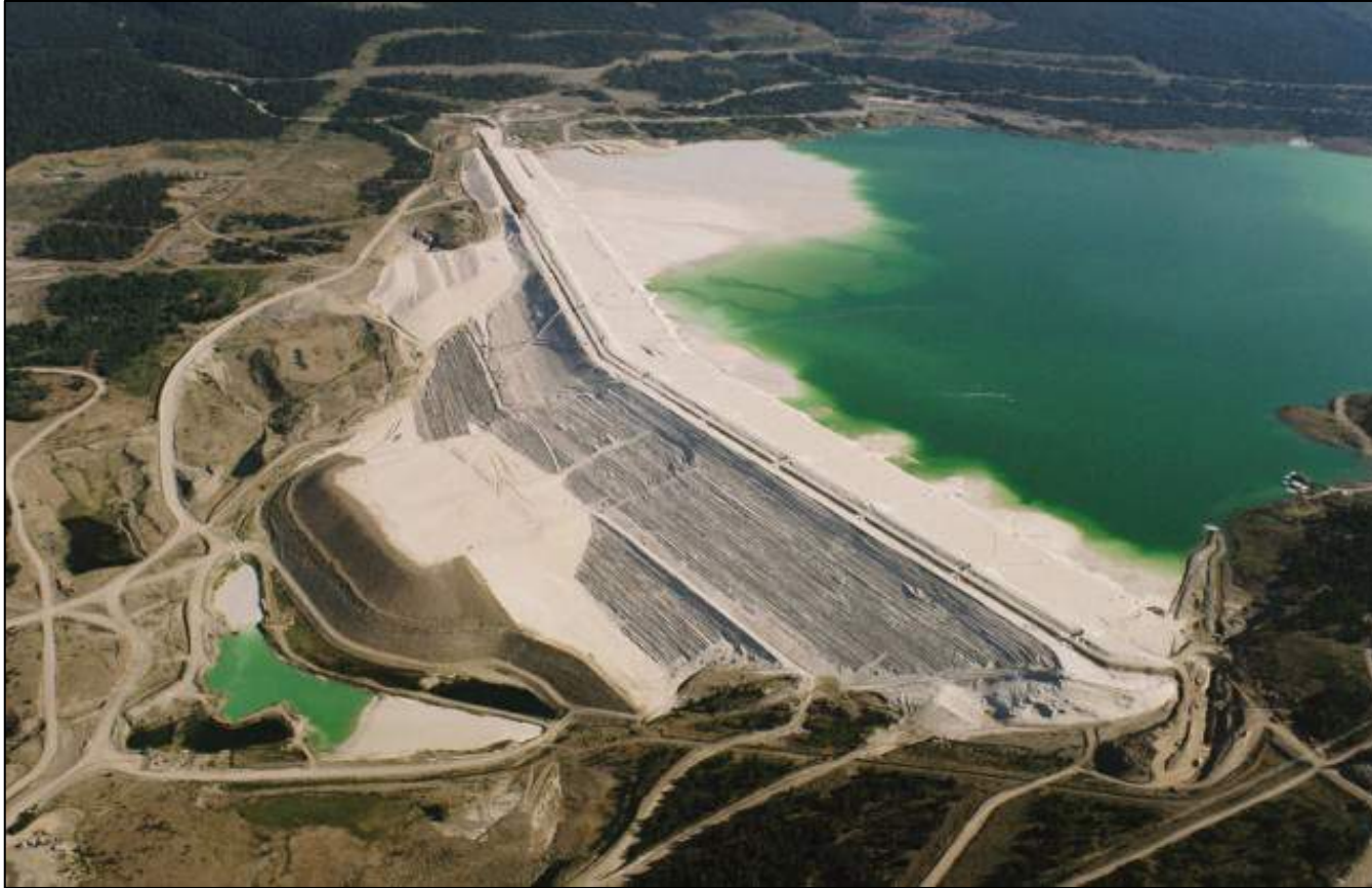
Highland Valley Copper Mine, Logan Lake, British Columbia, Canada
