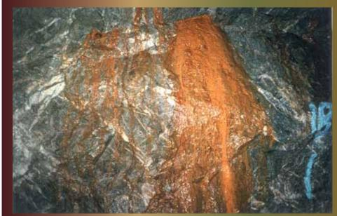
Figure 1: Acid drainage is red or orange because of the iron in it. Acid on tunnel walls at Kensington gold mine (Southeast Alaska). Photo - D. Chambers.
